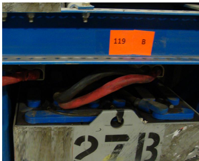
Clearly labeled battery using 3-digit organization
