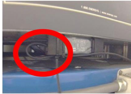
Correct Strain Relief Technique
